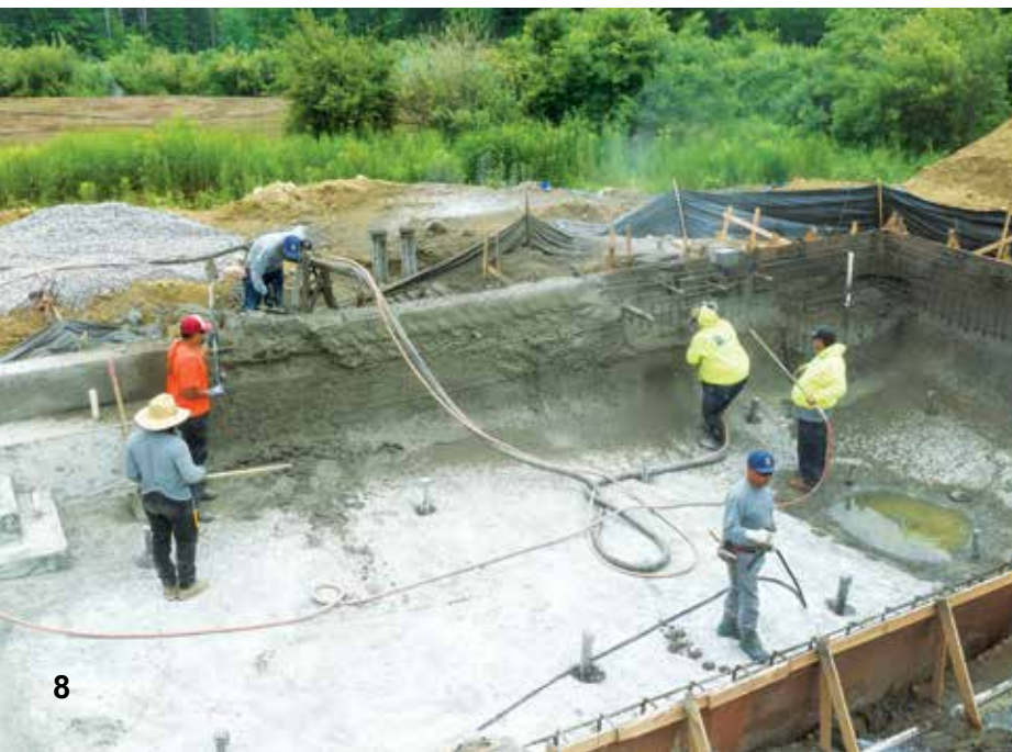
A crew sprays shotcrete to form a pool.
