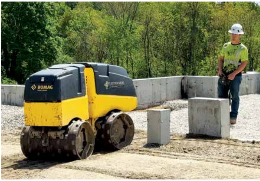
One of Earthworks' crew members remotely operates a BOMAG BMP 8500 compactor.
