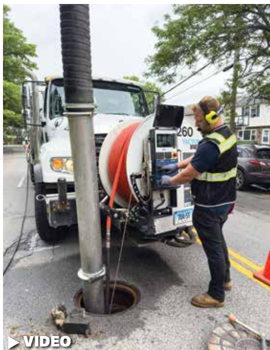
Liam Kenny operates a Vactor 2100i combination sewer cleaner via a control panel.
