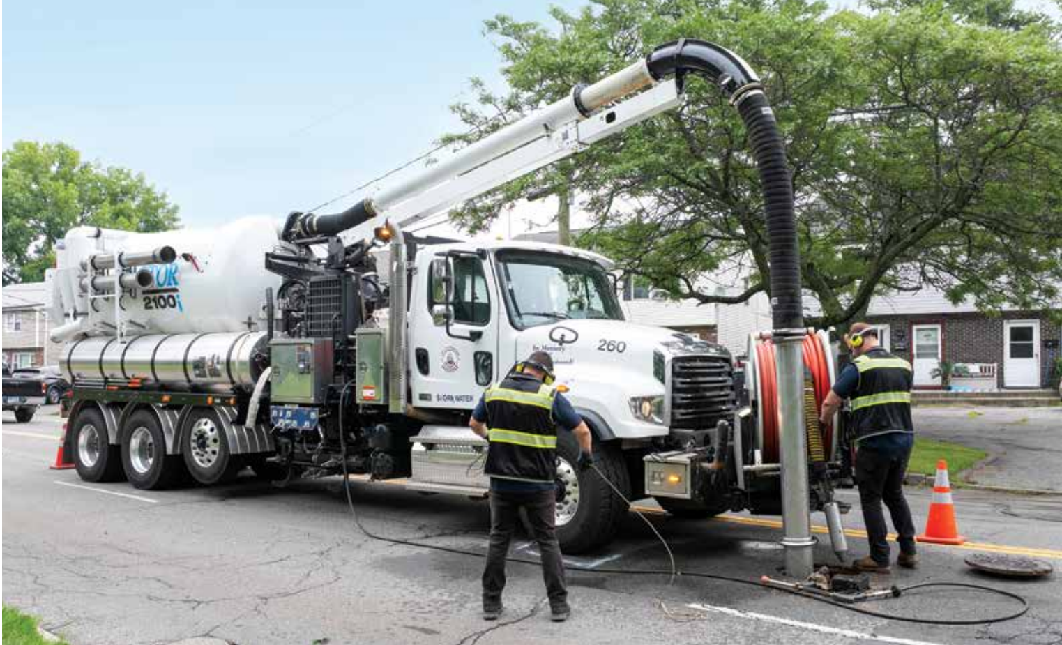
With a Vactor 2100i combination sewer cleaner, operators remove material from Stamford's storm drains.
