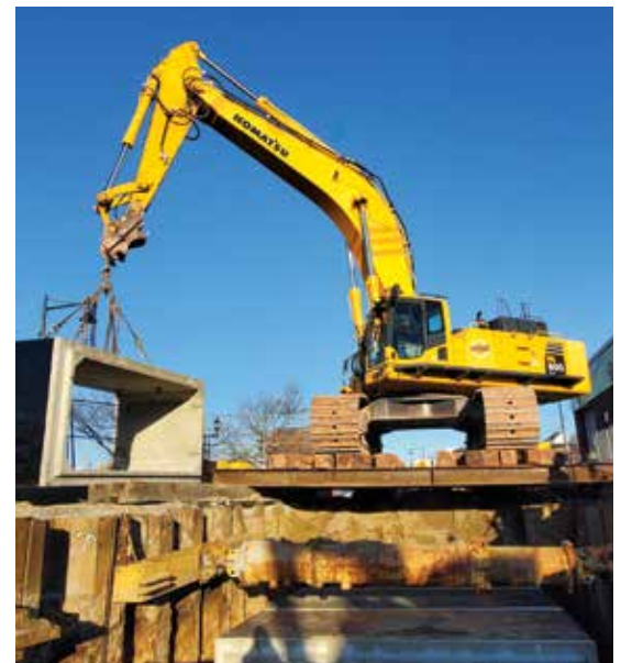
A Komatsu PC800 excavator was utilized to set large structures as part of a high-profile urban utility job site.
